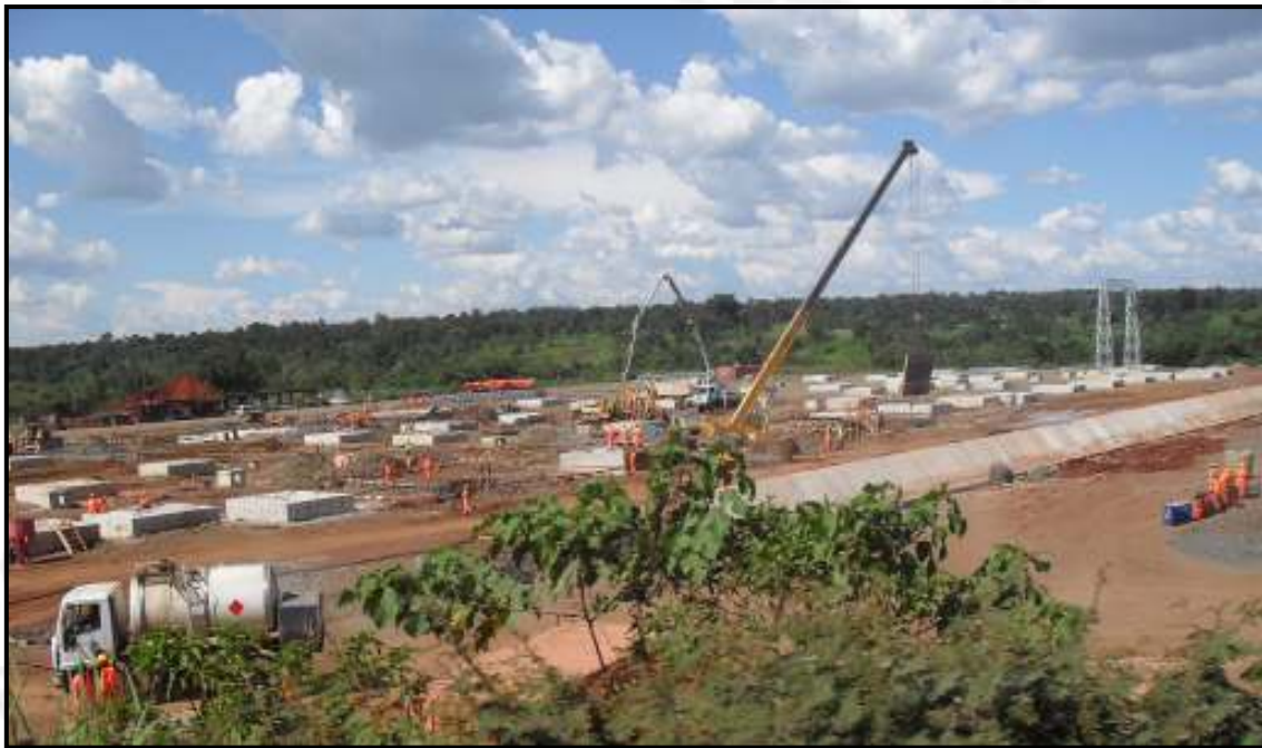
The Switchyard being Constructed - October 2009
